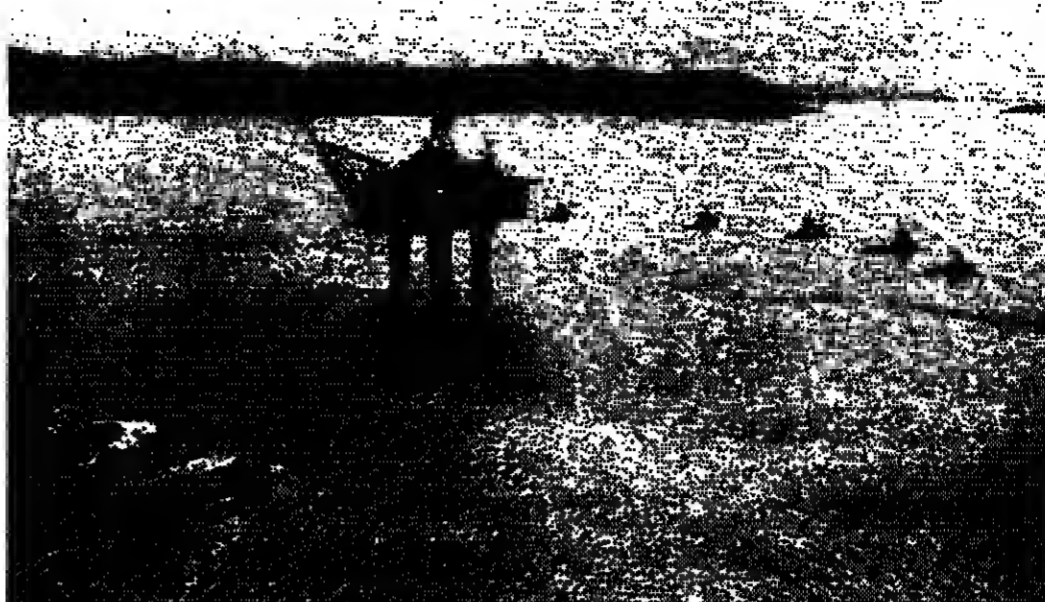
A fleet of eight tugboats moving the Statfjord-B oil platform to a drilling site in the North Sea.
